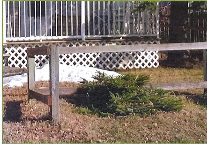
Figure 26. Example of lattice sheathing
