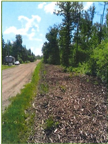
Figure 32. Mulched Ditches
